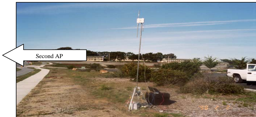
Figure IV-5. First ground AP. (Fort Ord mobile test JAN 2007).
